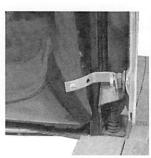
**6** Secure all four brackets to the shroud using 1 /2" No. 10 bolts and lock nuts
